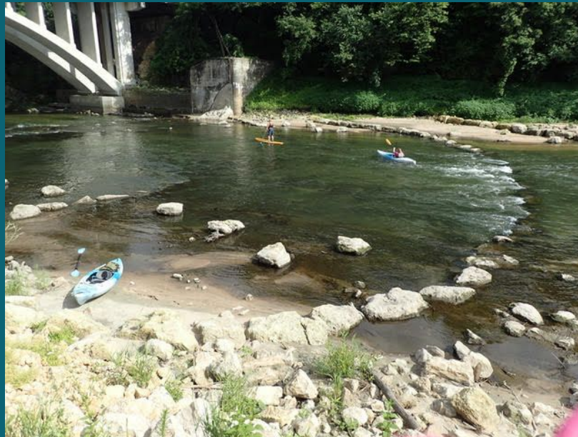
Photographs of rock riffle/pool restoration on Zumbro River near Oronoco
