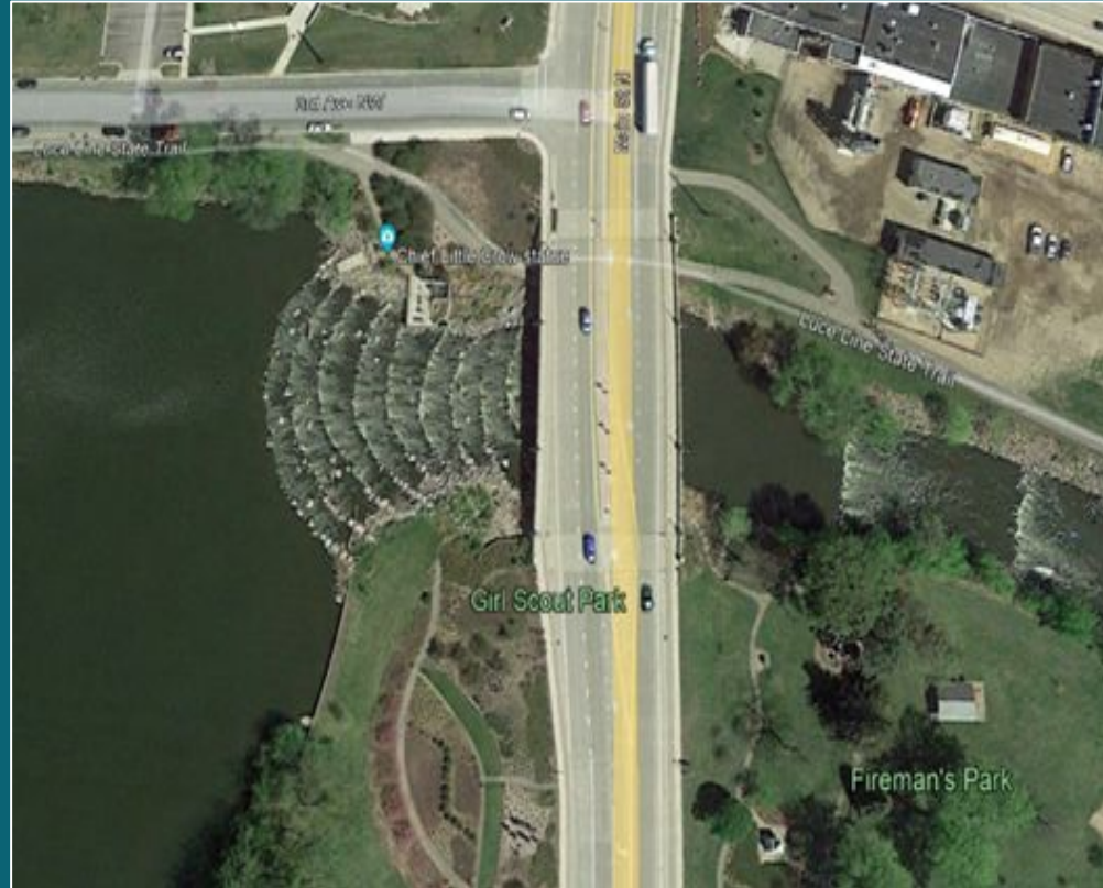
Aerial view of rock riffle/pool restoration, Crow River, City of Hutchinson
