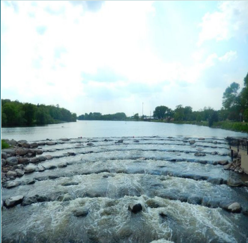
Looking upstream at rock riffle/pool restoration, Crow River, City of Hutchinson
